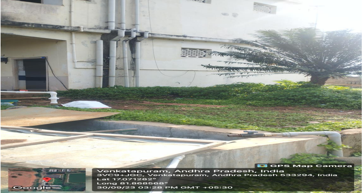
Rain Water Collection Tank
