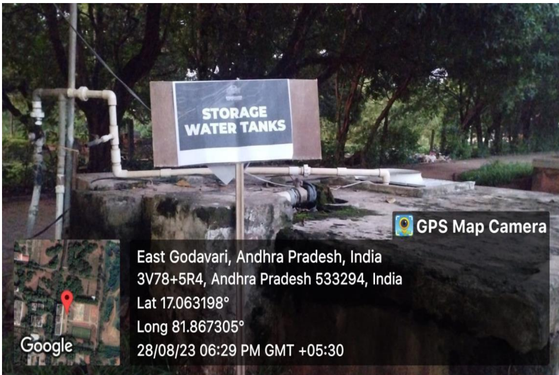
Closed Storage Tank
