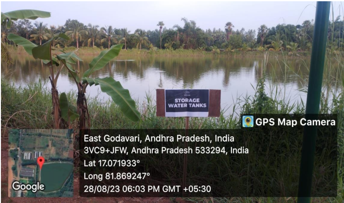
Open Storage Tank
