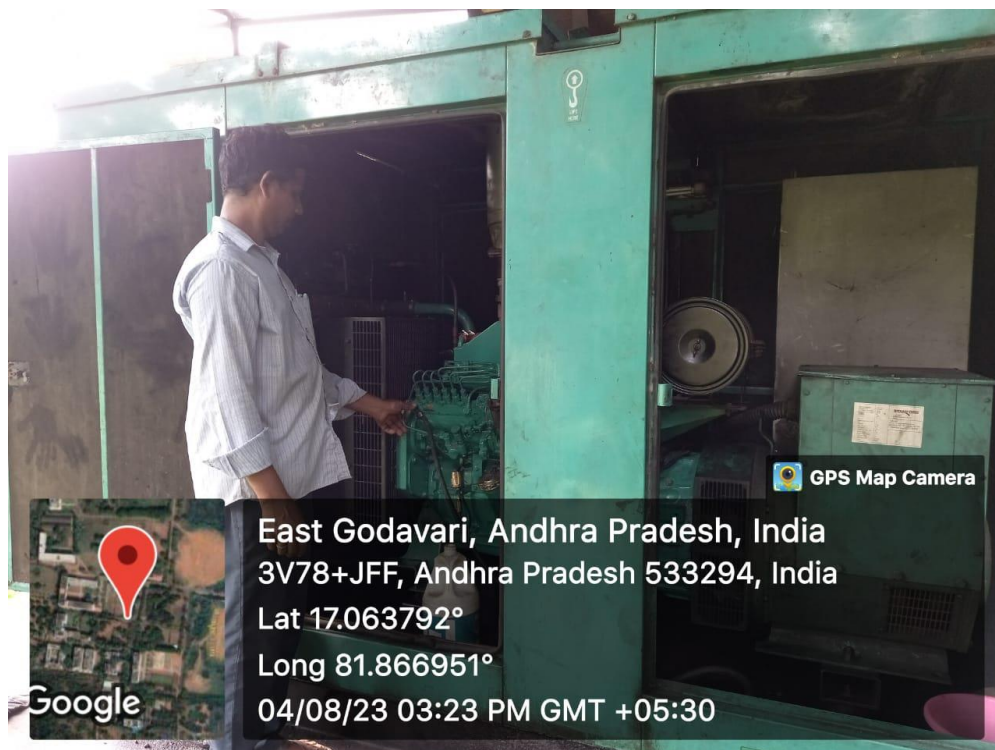
Maintenance of 125 kVA Generator at RK Block
