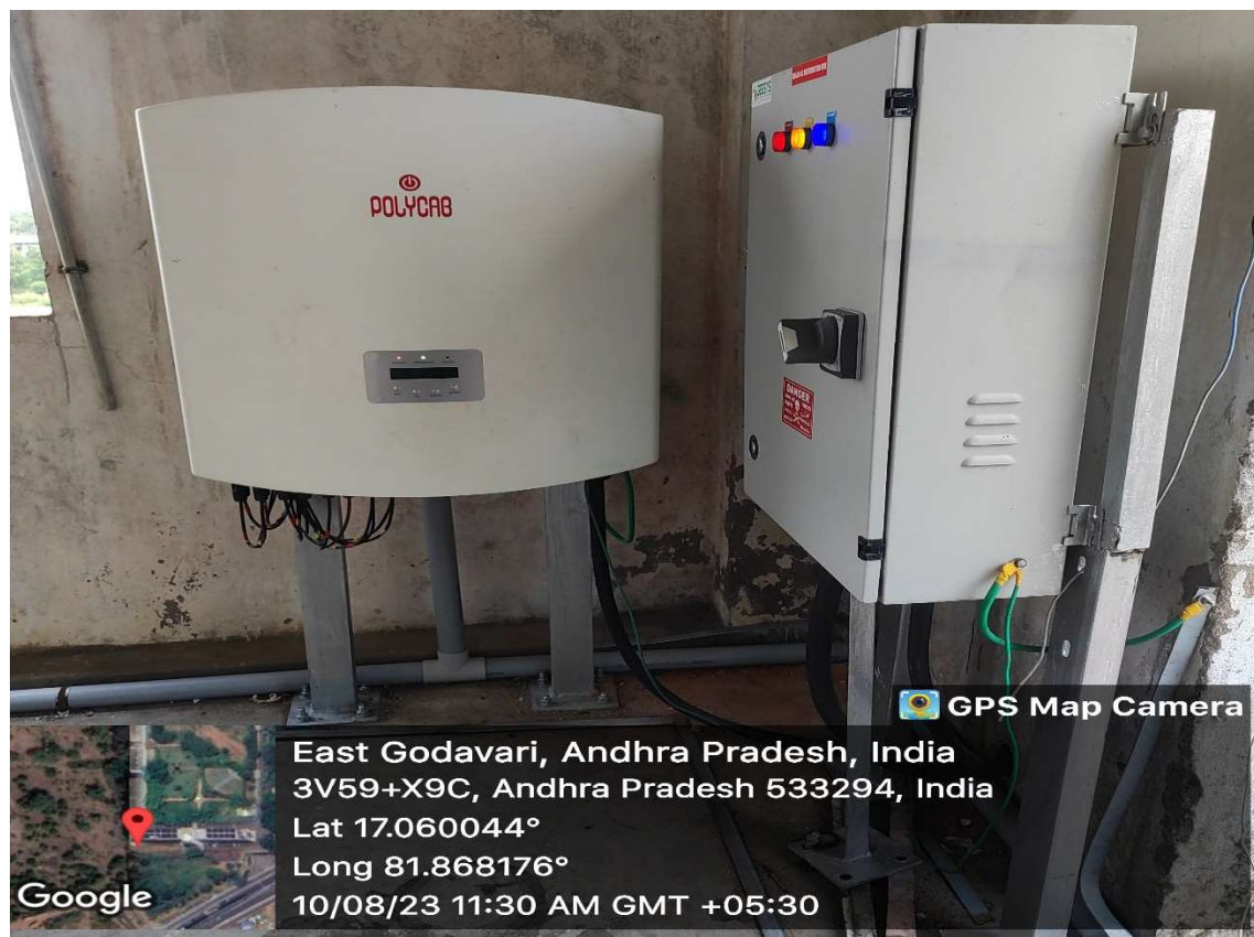
Inverter Setup @ Visvesvaraya Block
