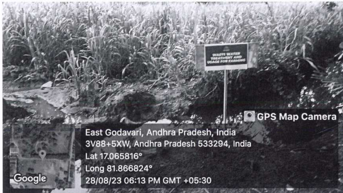
Diversion of waste water through open drainage system
