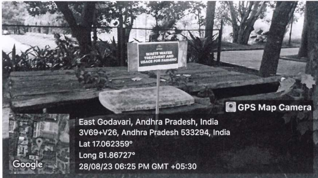
Storage of waste water in closed tank
